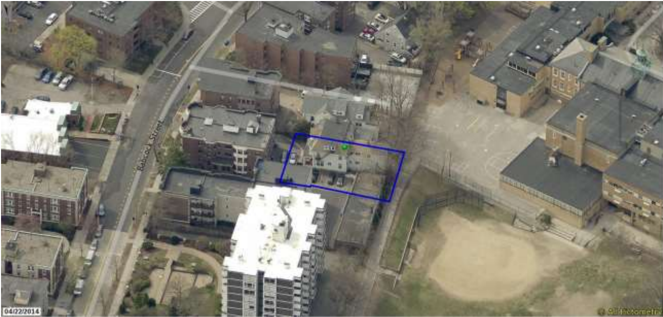
Aerial view of 46 Babcock Street, looking south.
