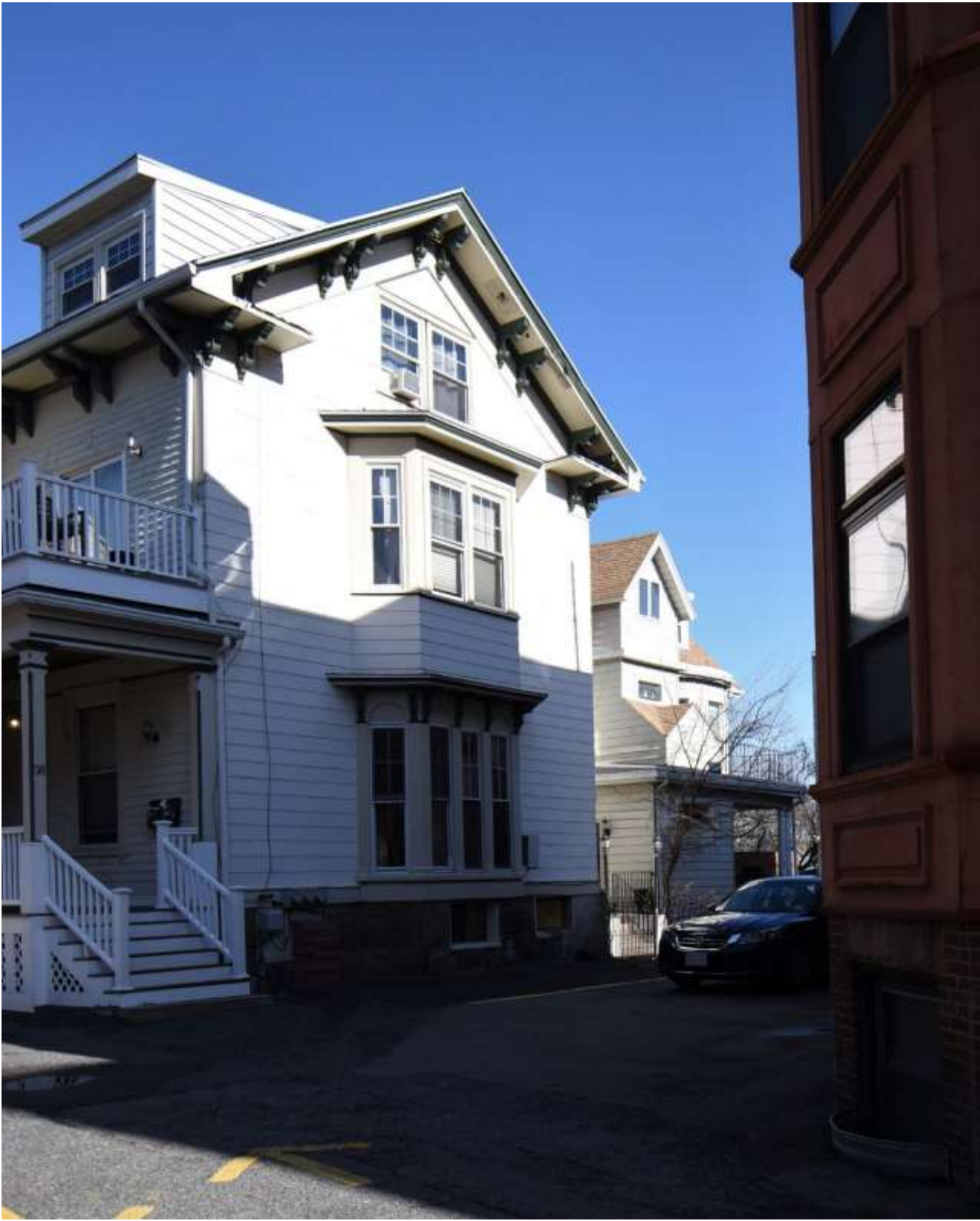
View from right, showing 46 Babcock behind neighbors 38 & 40 Babcock Street
