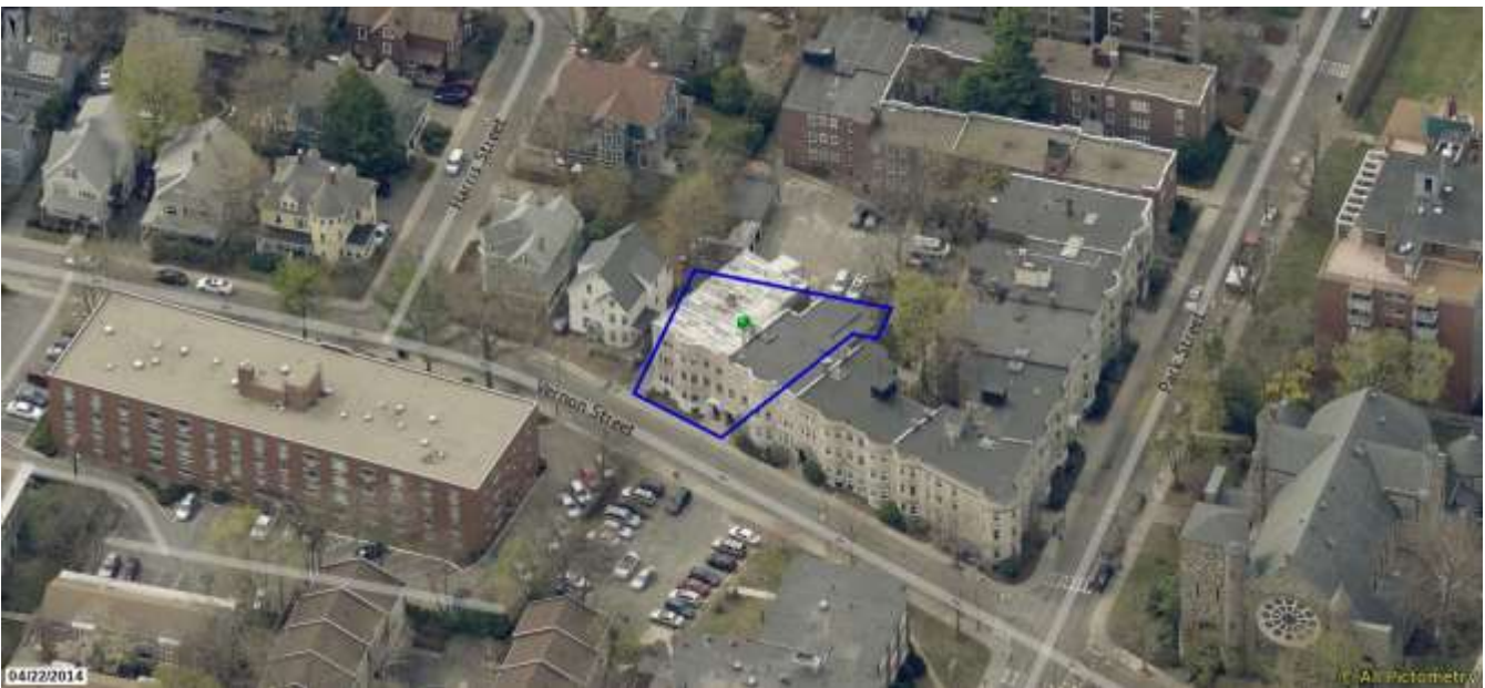
Aerial view of 50 Vernon Street, looking south.
